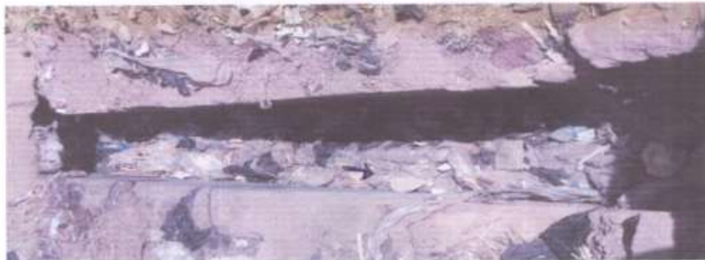
Plate 8: Showing drainage channels blocked with solid waste in the study area.
